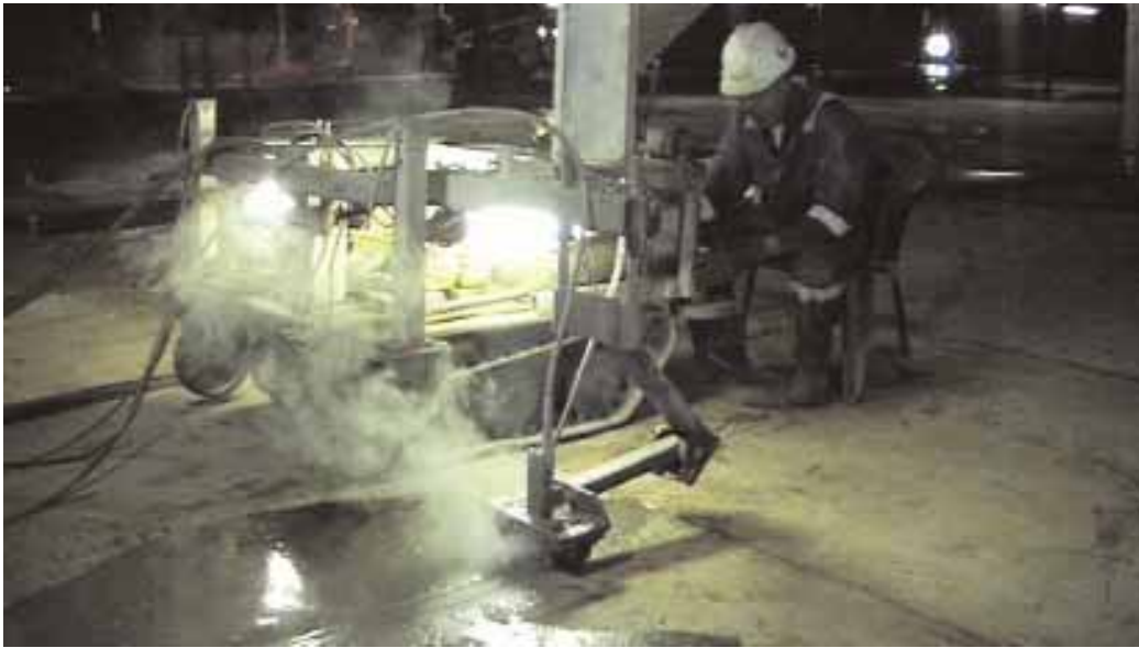
Directing cutting operations inside the tank
