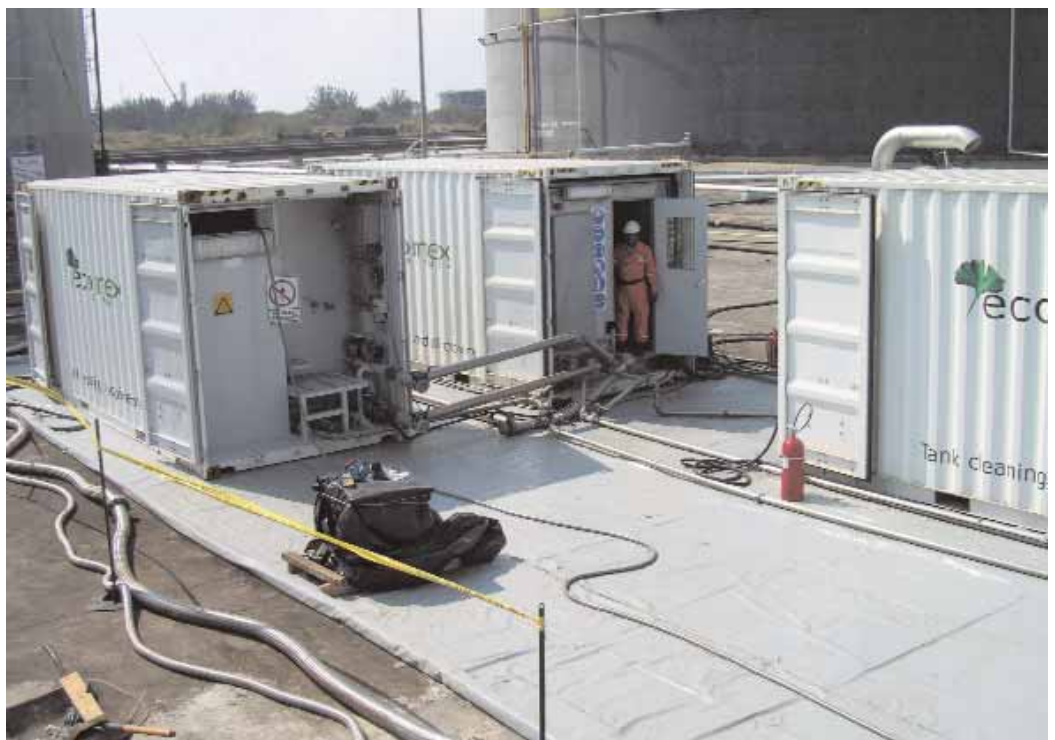
Blabo equipment on site in Mexico
